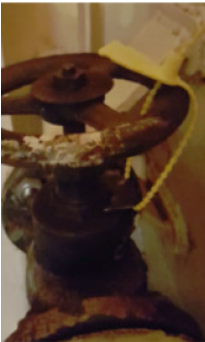
Correctly applied seals, the seal will break in case the valve or flange is opened.
