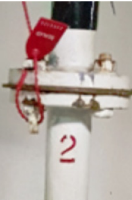
Correctly applied seals, the seal will break in case the valve or flange is opened.
